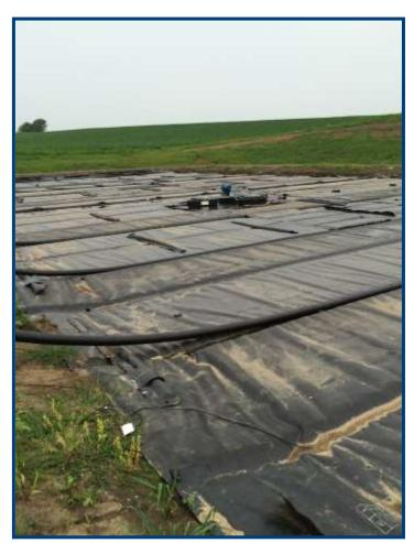
to handle a design flow of 0.098 MGD. Each lagoon is divided into three cells using Lemna's LemTec<sup>™</sup> Reverse Miter Hydraulic Baffle, which is custom designed to minimize short-circuiting between each cell. The lagoons are covered with Lemna's
