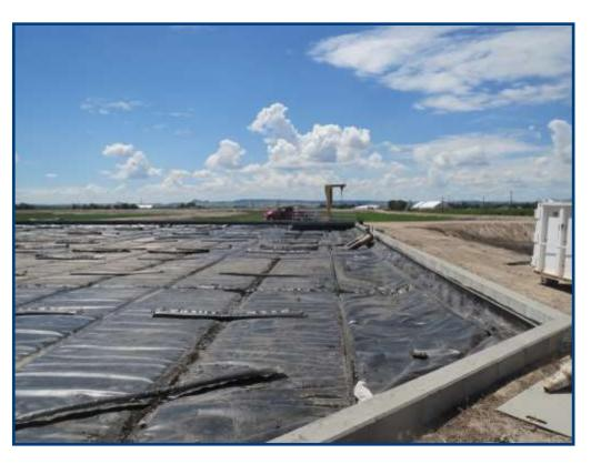
the design of the cover system makes operational and maintenance activities such as vegetation removal easier, more manageable and less reliant on heavy equipment. With a 20 year life expectancy, the LemTec<sup>™</sup> Modular Insulated Cover will provide years of service.
